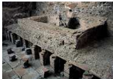
Hypocaust in the Stabian Baths. Notice the floor suspended on brick piles, so that hot air can circulate beneath and warm both the room and the tank of water for bathing.
