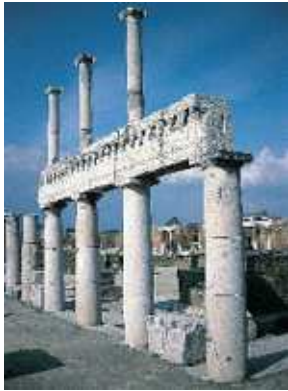
Part of the colonnade, which had two stories, seen from inside. You can see the holes for the floor beams of the top story.
